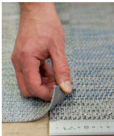
FLOW 1. Overlap 2 sheets of flooring 4 cm and double cut.
