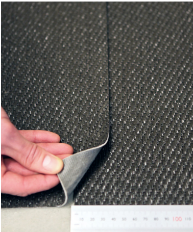
BKB 1. Overlap 2 sheets of flooring 4 cm and double cut.
