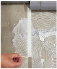
**5.** Glue the subfloor and remove the masking tape while still reachable.
