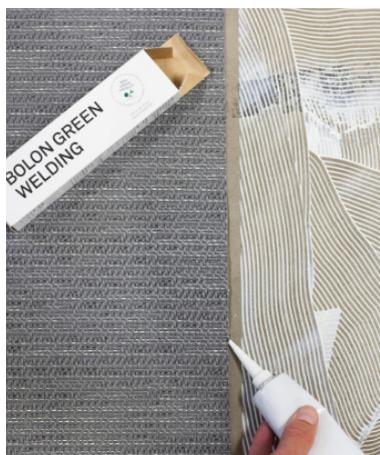
7. Add Bolon Green Welding along the cross-section area of the sheet. Avoid overflow on floor covering surface.
