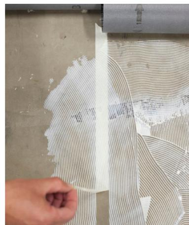
5. Glue the subfloor and remove the masking tape while still reachable.
